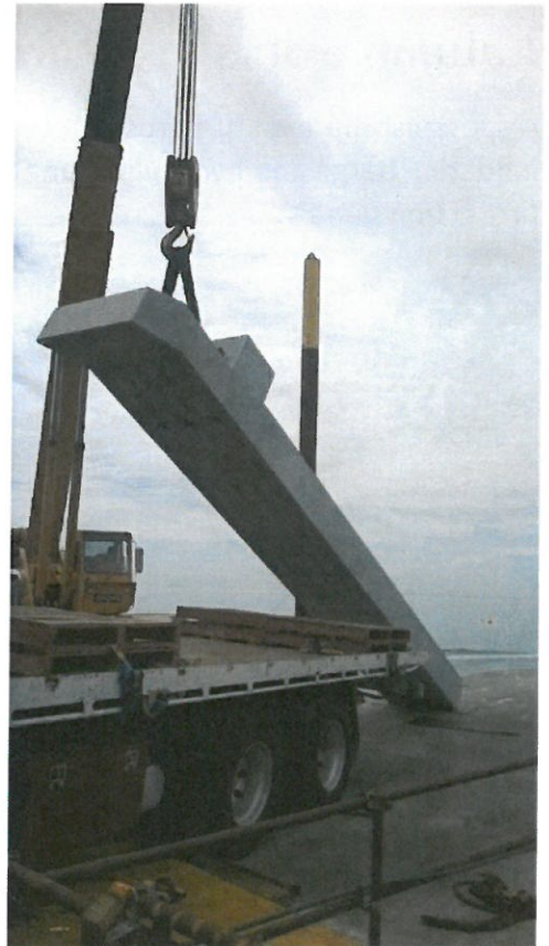
Wave panel being delivered to the pier
