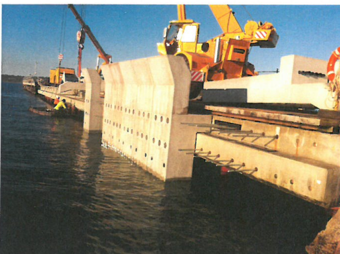
Wave panels being installed on the edge of the pier
