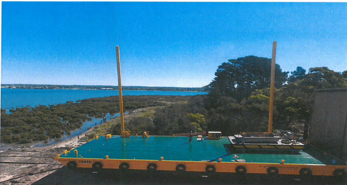
Barge to be used to remove damaged wave panels
