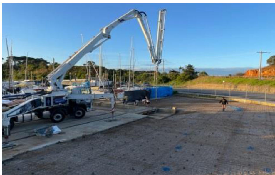
Above Photo: Concreting the yard
